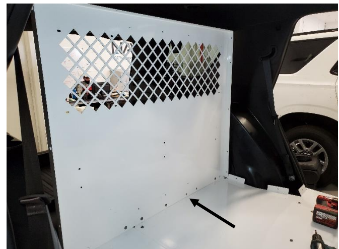
Attach rear bulkhead to floor using 1/4" x 3/4" Phillips head bolts and flat washers.
